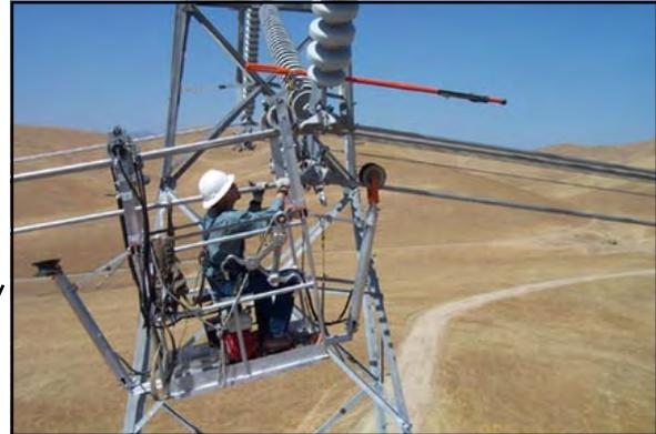
Leading wheel has taken the load and leading pair of drive wheels have been moved to the side to allow cart to pass insulators.
